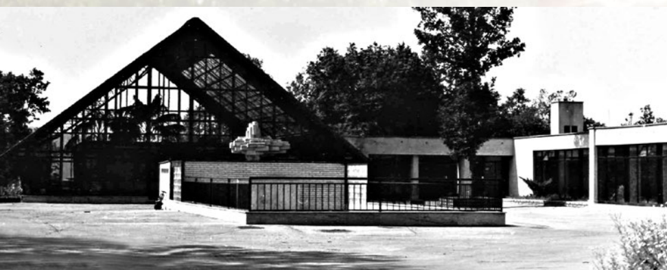
The vivarium completed in 1972 was constructed from a glazed hall with a gable roof and a ground floor corridor
